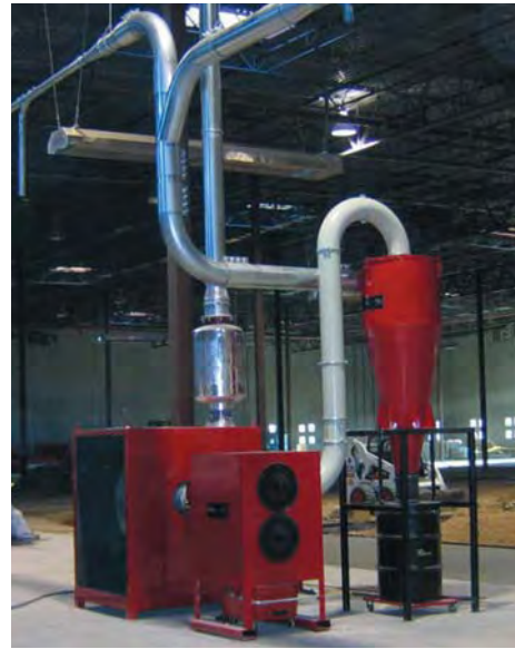
Above: FA2000 Filtration System as part of a central vacuum system, complete with a High Efficiency Cyclone pre-separation system.
